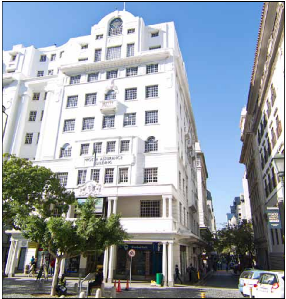
PROTEA HOUSE, CAPE TOWN
