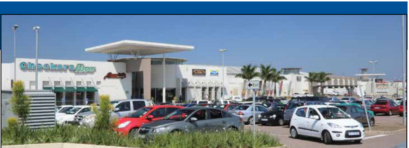
THE RIDGE@SHALLCROSS, SHOPPING CENTRE, CHATSWORTH, DURBAN
